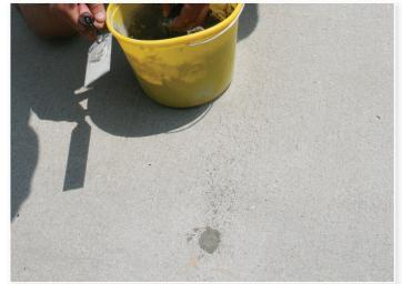
**Step 4**The drilled holes are patched and smoothed over
