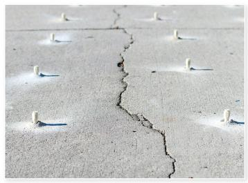
**Step 2**Temporary injection ports are installed
