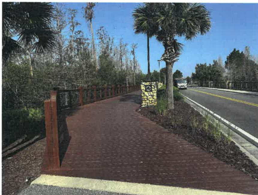
Photo 2. South approach of boardwalk, looking North
