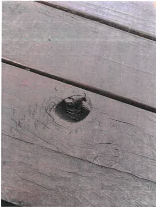
Photo 5. Knot in decking
